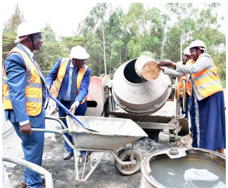
Vice-Chancellor Prof. Joyce Agalo pours the concrete mixture into the mixer during the launch of the construction works, accompanied by Chair of Council Dr. Peter Maangi Mitiambo (left, with the wheelbarrow) and Safaricom PLC General Manager for the Coast and Eastern Region, Jackson Mutua.
